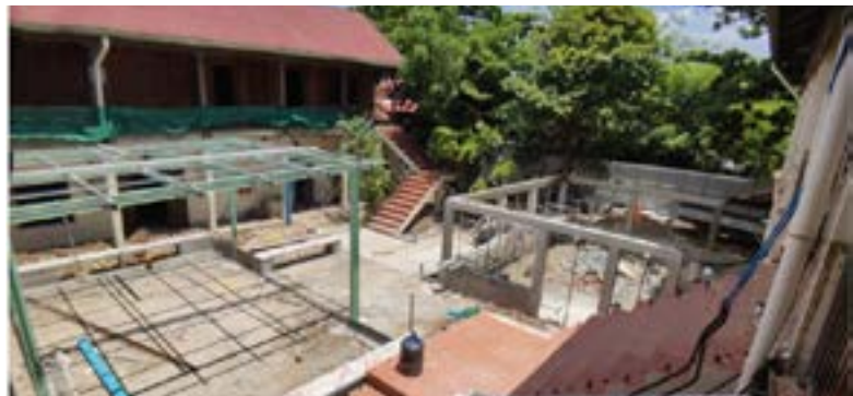
Progress to 17th June 2020
