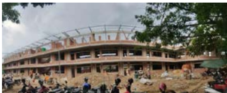
Progress to 20th July 2020
