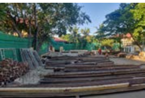
Dismantling the buildings
