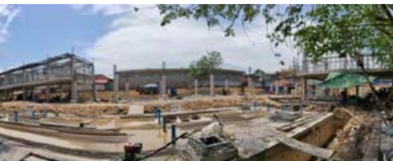
Progress to 27th April 2020
