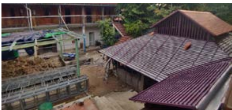
Progress to 28th August 2020
