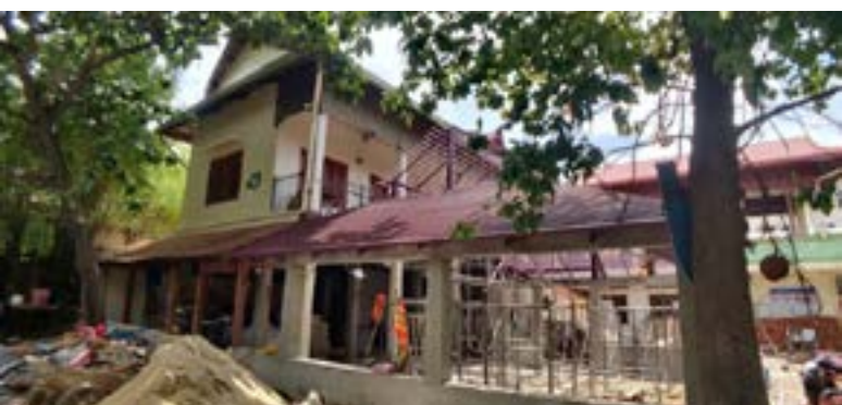
Progress to 13th August 2020
