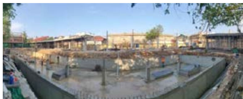
Progress to 14th April 2020
