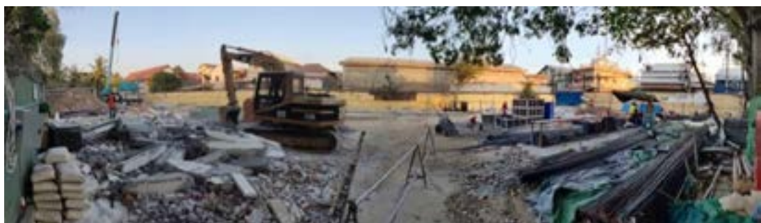
Demolition of the buildings
