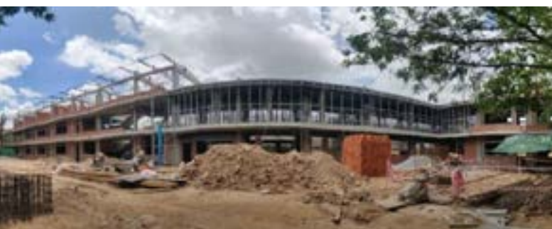
Progress to 15th June 2020
