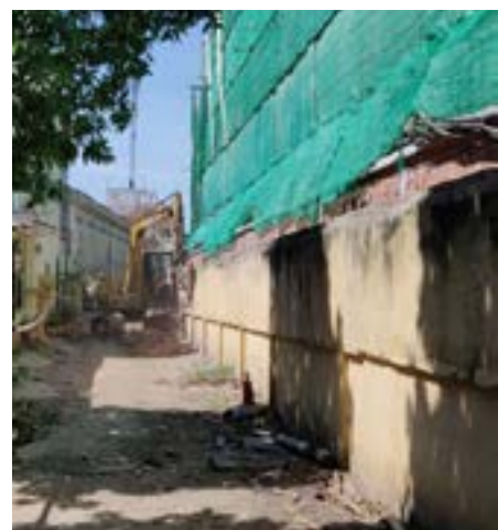
Building a new surrounding wall
