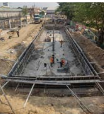
Building a retention basin
