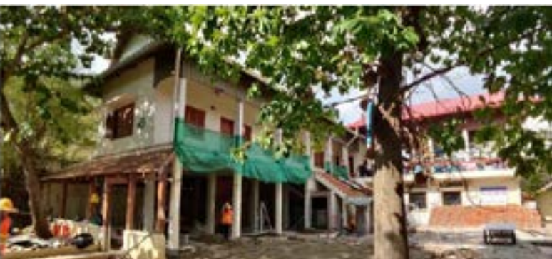
Progress to 22nd May 2020
