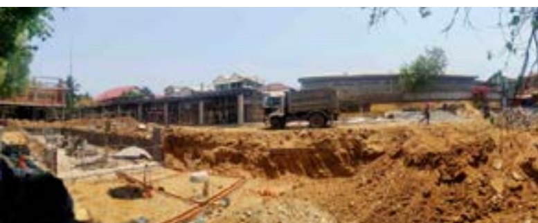
Laying the foundations
