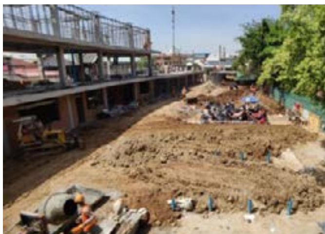
The backfill of the retention basin was completed in May 2020
