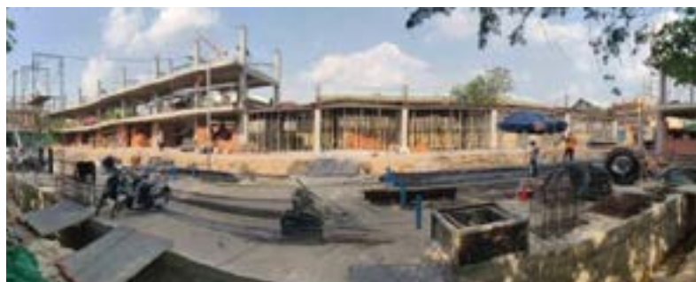
Progress to 15th May 2020
