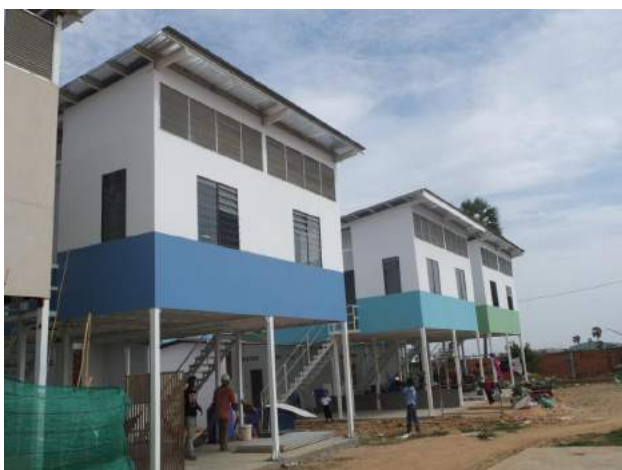
Second phase of construction, Houses delivered in July 2015
